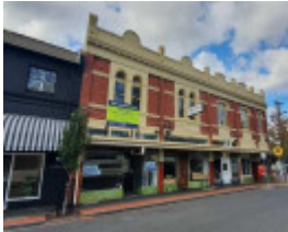
11-15 Beatty Avenue, Armadale
