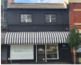
16-17 Beatty Avenue, Armadale
