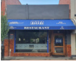
22 Beatty Avenue, Armadale
