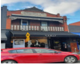
23 Beatty Avenue, Armadale
