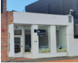
25 Beatty Avenue, Armadale
