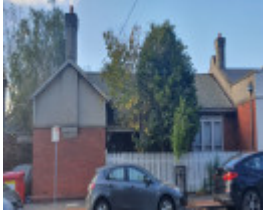
34 Beatty Avenue, Armadale
