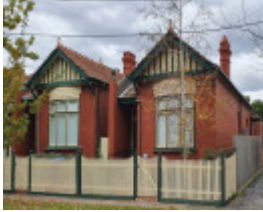
2 Densham road, Armadale
