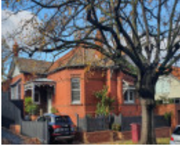
14 Densham Road, Armadale
