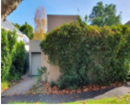
35 Densham Road, Armadale
