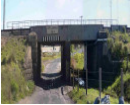
Melbourne-Geelong Railway Bridge and Stone Ford, Hobsons Bay Heritage Study 2006
