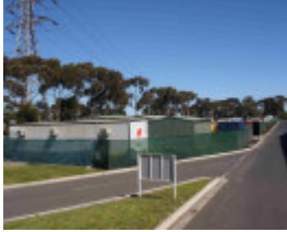
Main Outfall Sewer, Hobsons Bay Heritage Study 2006
