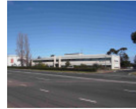
Standard Vacuum Refining Co. Complex (former), Hobsons Bay Heritage Study 2006 - Administrative building (Pegasus Centre) designed by Stephenson & Turner and constructed c.1955
