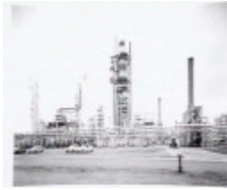
Standard Vacuum Refining Co. Complex (former), Hobsons Bay Heritage Study 2006 - c.1955 view showing Thermoform Catalytic Cracker in centre.
