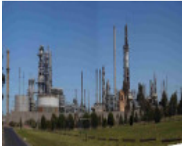
Standard Vacuum Refining Co. Complex (former), Hobsons Bay Heritage Study 2006
