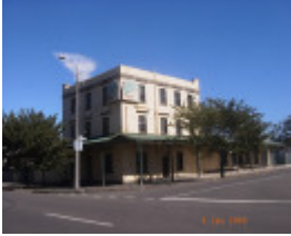
Oriental Hotel (former), Hobsons Bay Heritage Study 2006
