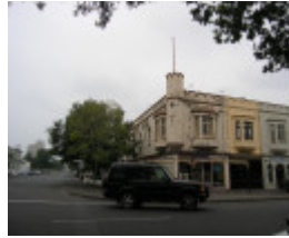
Craigantina, Hobsons Bay Heritage Study 2006
