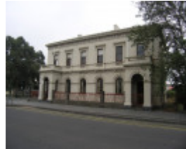
Customs House (former), Hobsons Bay Heritage Study 2006
