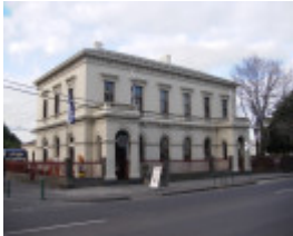
Customs House (former), Hobsons Bay Heritage Study 2006
