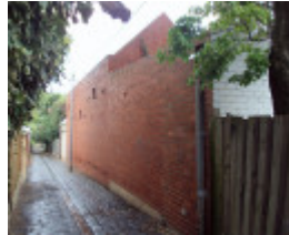
Stables at the rear of 64 Rose Street, Armadale.
