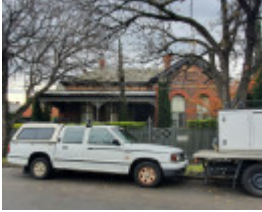
1 Royal Crescent, Armadale
