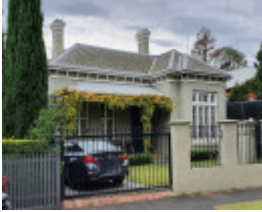
3 Royal Crescent, Armadale
