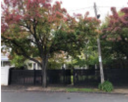
6 Royal Crescent, Armadale
