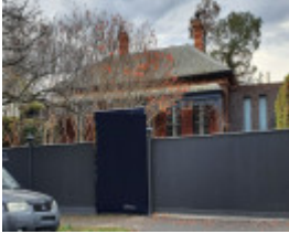
7 Royal Crescent, Armadale
