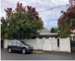
8 Royal Crescent, Armadale
