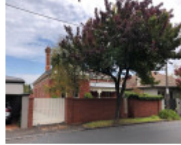
12 Royal Crescent, Armadale
