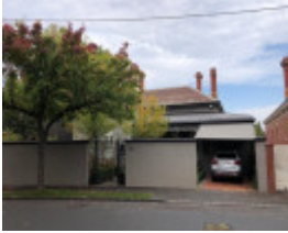
14 Royal Crescent, Armadale
