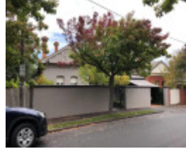
14 Royal Crescent, Armadale
