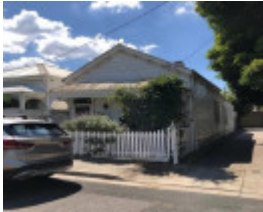
1 Watson Street, Armadale
