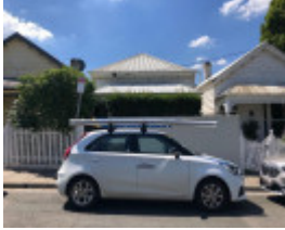
2 Watson Street, Armadale
