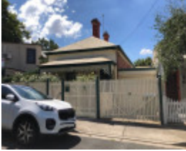
7 Watson Street, Armadale
