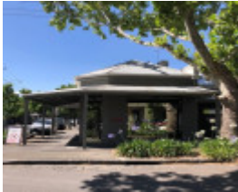
1 Davis Avenue, South Yarra
