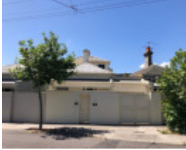
7 Davis Avenue, South Yarra
