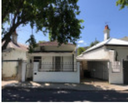
11 Davis Avenue, South Yarra
