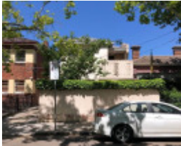
20 Davis Avenue, South Yarra
