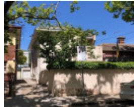
20 Davis Avenue, South Yarra
