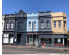
338-344 Punt Road, South Yarra
