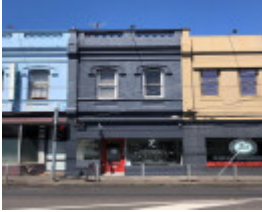
340 Punt Road, South Yarra
