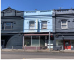
342 Punt Road, South Yarra
