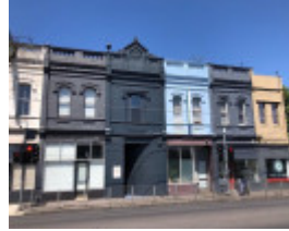
338-344 Punt Road, South Yarra
