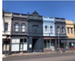
338-346 Punt Road, South Yarra
