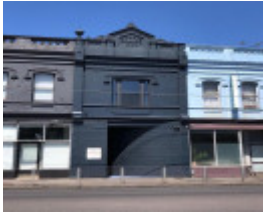
344 Punt Road, South Yarra
