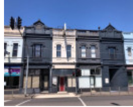
344-350 Punt Road, South Yarra
