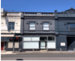
346 Punt Road, South Yarra
