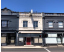
348 Punt Road, South Yarra
