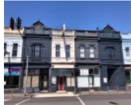
344-350 Punt Road, South Yarra
