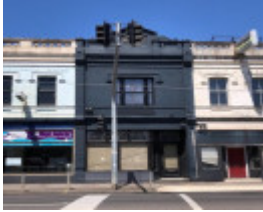
350 Punt Road, South Yarra
