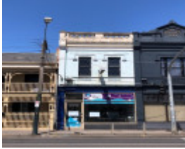
352 Punt Road, South Yarra
