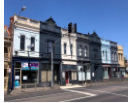
338-352 Punt Road, South Yarra
