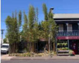
360 Punt Road, South Yarra
