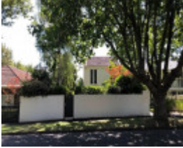
3 Belson Street, Malvern East
