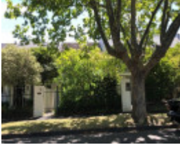
5C Belson Street, Malvern East
