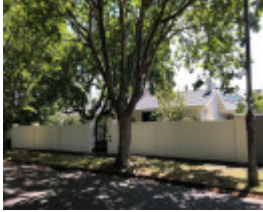
7 Belson Street, Malvern East
