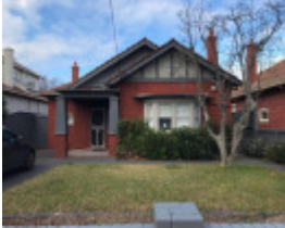
22 Belson Street, Malvern East
