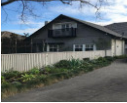
29 Belson Street, Malvern East
