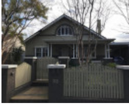
33 Belson Street, Malvern East
