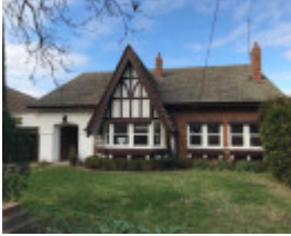
36 Belson Street, Malvern East
