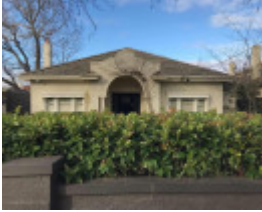
40 Belson Street, Malvern East
