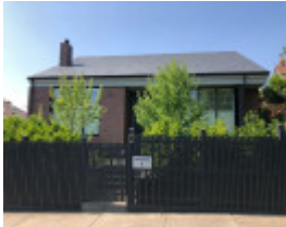
1 Central Park Road, Malvern East
