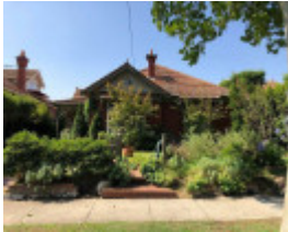
7 Central Park Road, Malvern East
