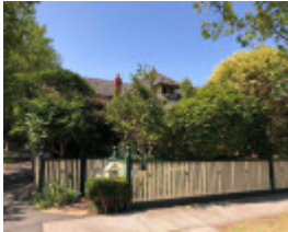
15 Central Park Road, Malvern East
