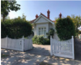
17 Central Park Road, Malvern East
